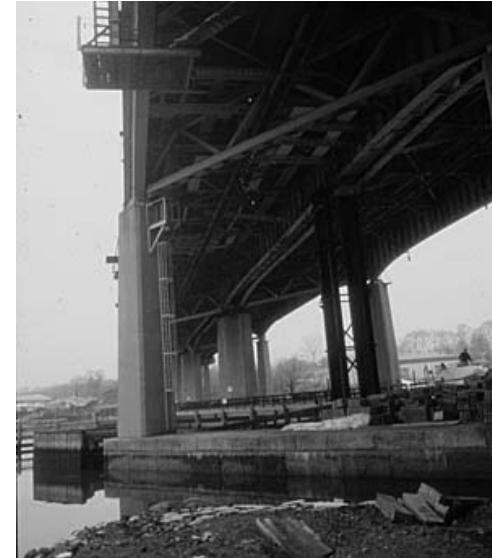
Reconstruction of the Mianus River Bridge, January 1984
