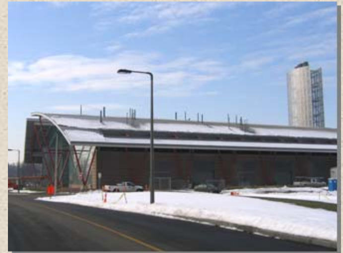
Central Heating Plant
