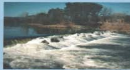
Union City Dam - Before
