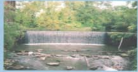
Bray's Buckle Dam
